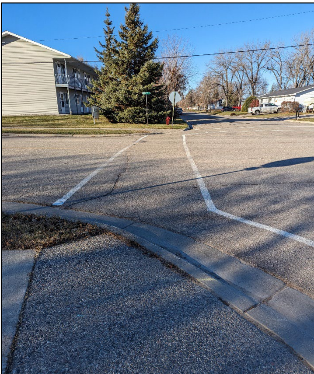
Barrette St./3rd St. NE Intersection - View Showing Apartment Building, Lack of Pedestrian Ramp & Lack of Sidewalk/Street Signage
